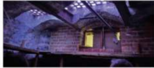
Existing vaults provide a character unique to Lewiston.
